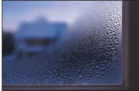
Condensation on the inside of a window-pane.
